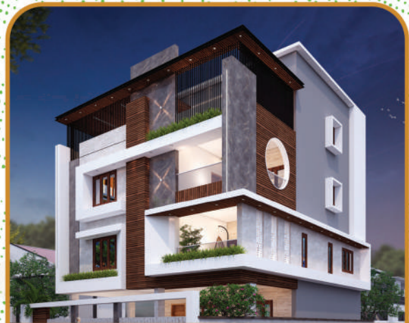
Ranjitha enclave Plot No 27, 7 cross street, Kamarajar nagar Perungudi 96
